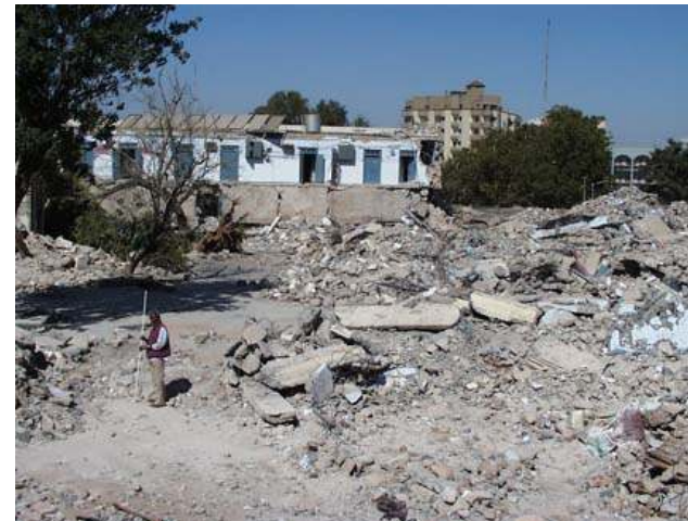
Photograph of the collapsed hospital (circled white in the left image)
